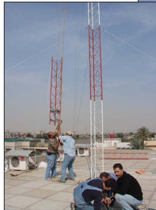
The new 150' 500kw tower goes up in Baghdad.
