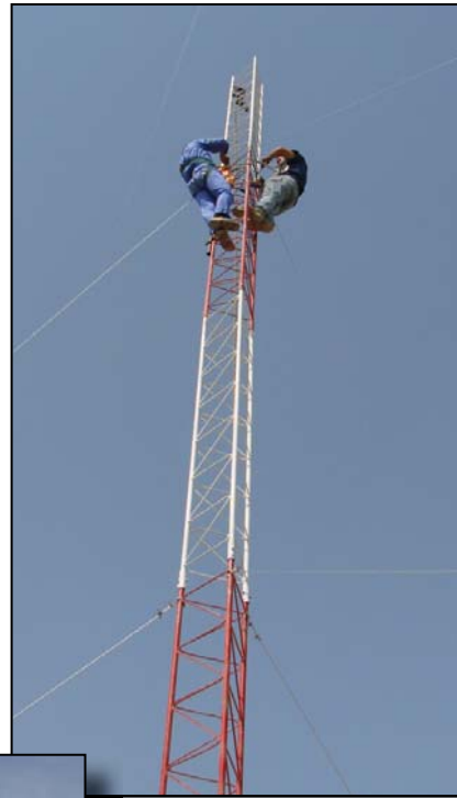
The new 150' 500kw tower goes up in Baghdad.
